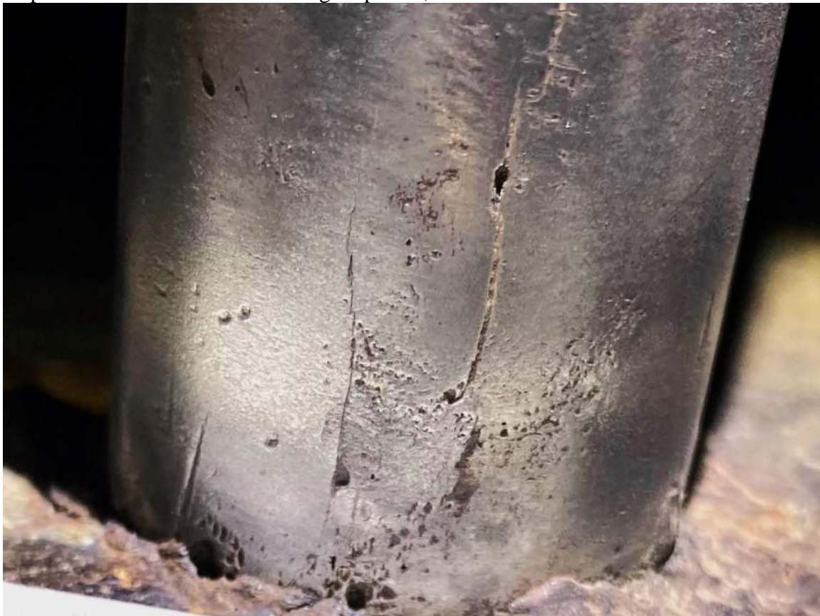
Inspection of stainless steel hanger rods in Hawaii's Wilson Tunnel
