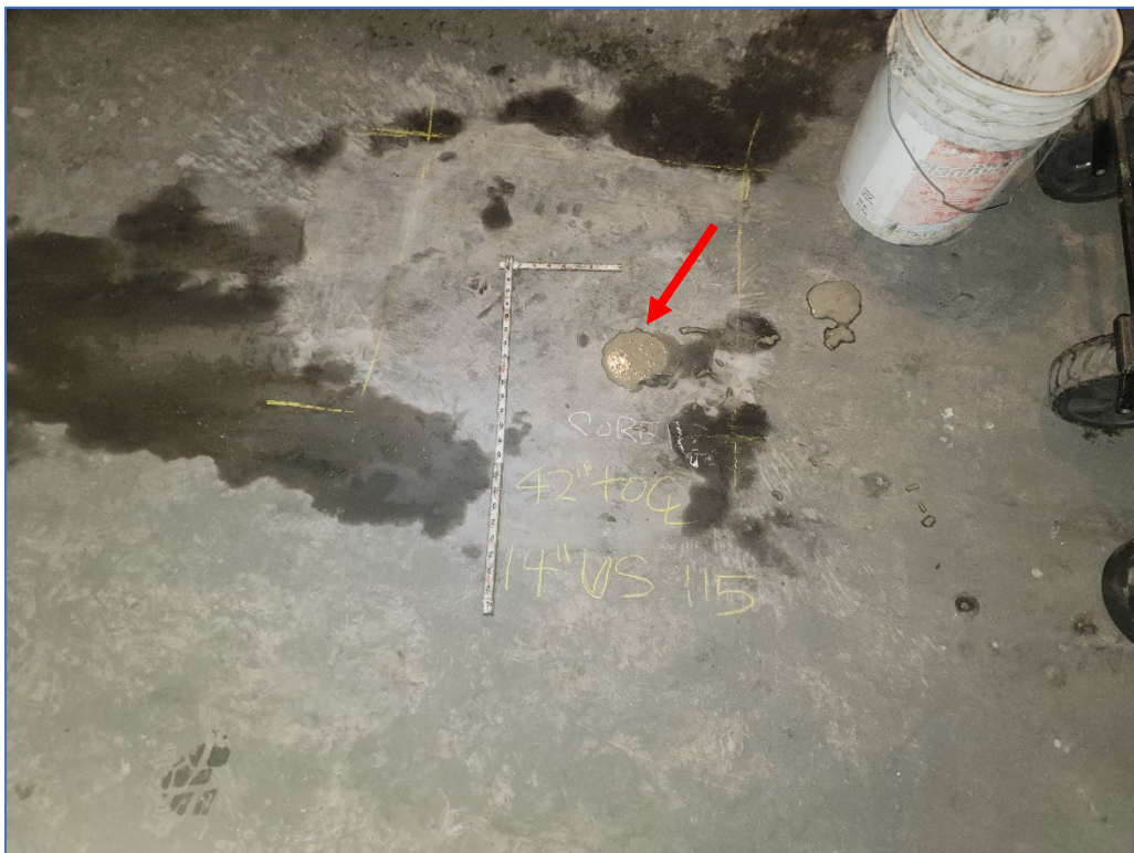
Photo 4: Typical core hole filled with cementitious grout (Core 11 shown).
