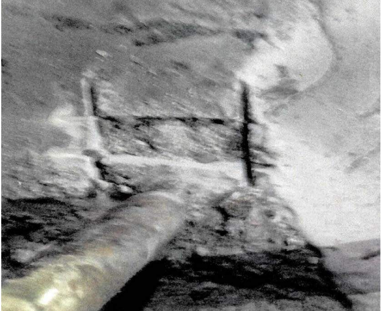
Figure 32. Rod #40 OB - Wilson Tunnel
