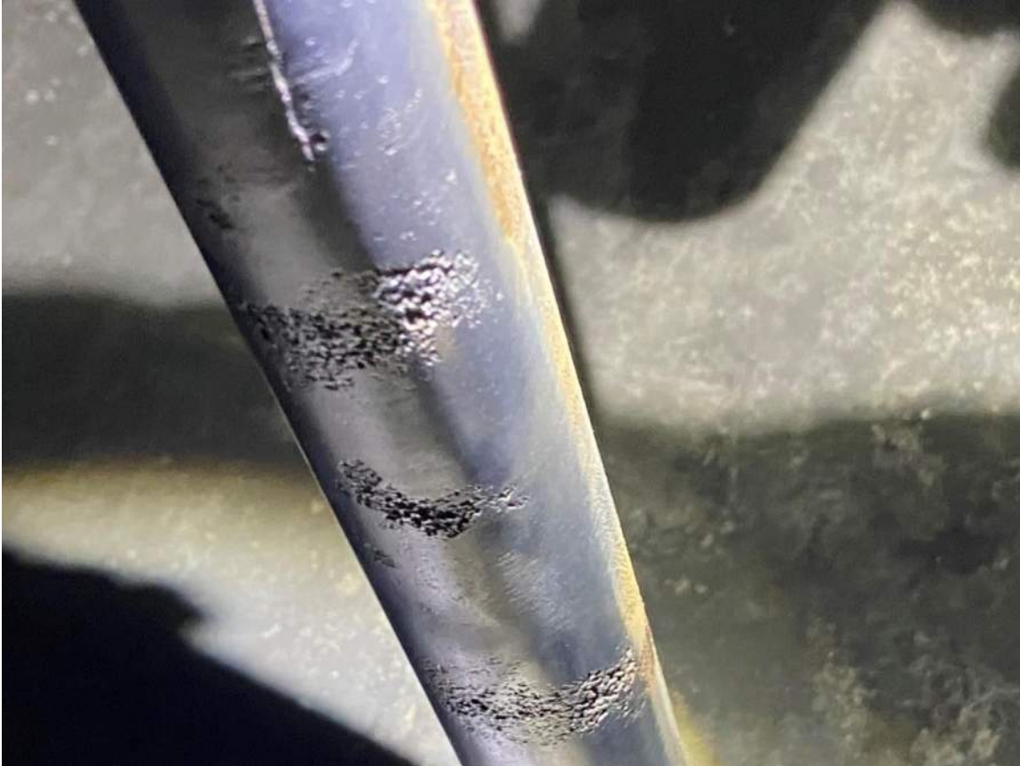
Severity level 3, visible cracking, and severe pitting
