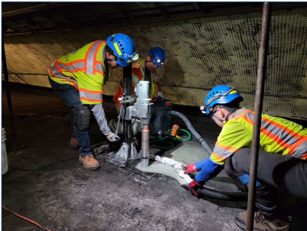
Photo 2: Core sample collection.
