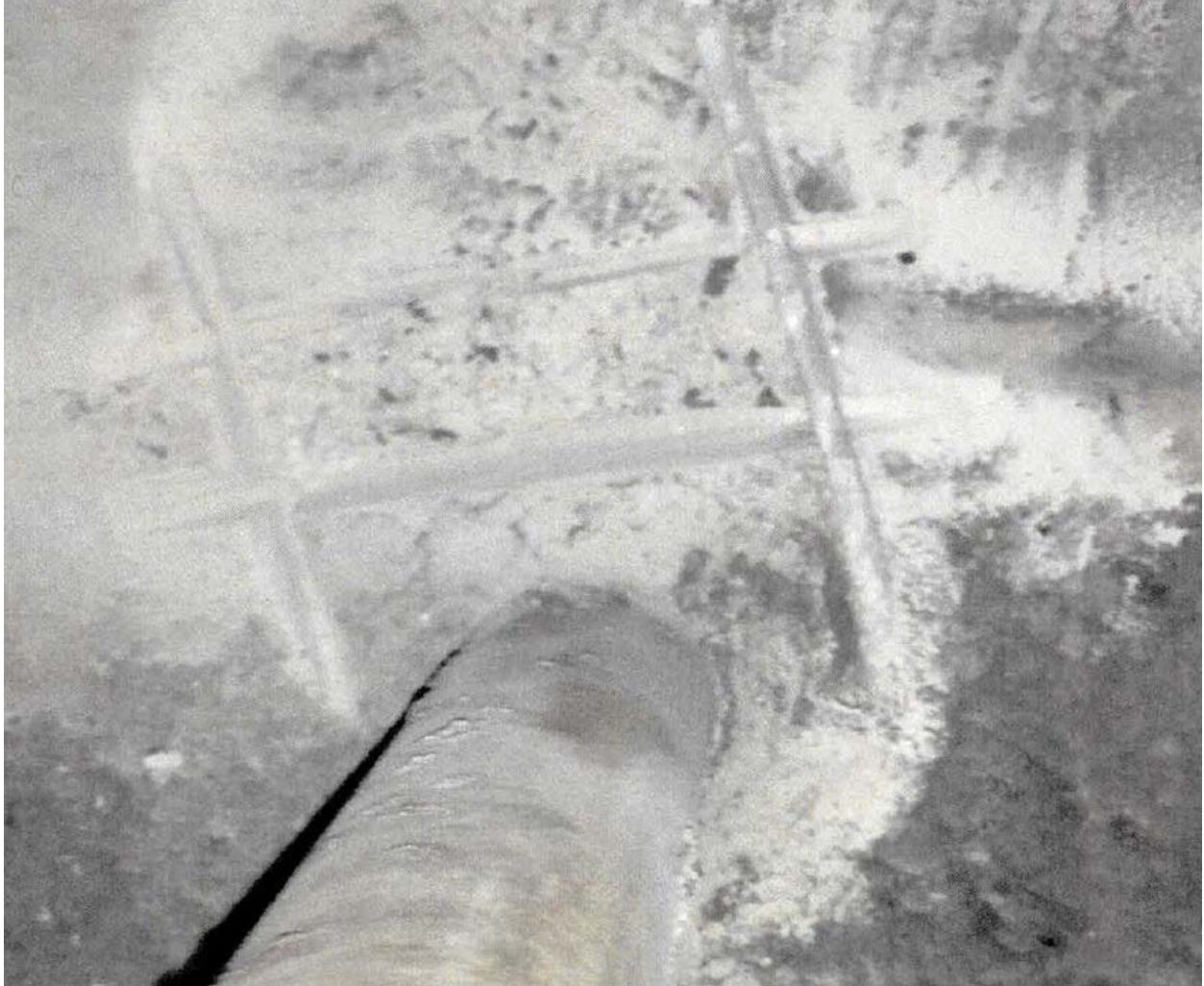
Figure 31. Rod #18 - Outbound (OB) Wilson Tunnel
